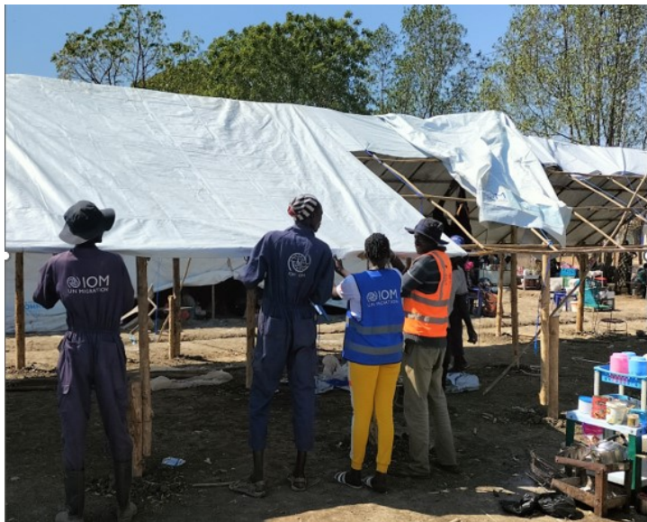
Construction of tents for new arrivals, Malakal © IOM South Sudan 2024
